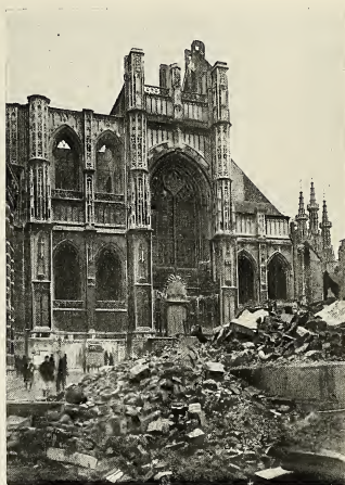
Louvain. Church of St. Peter The western wing after the fire
